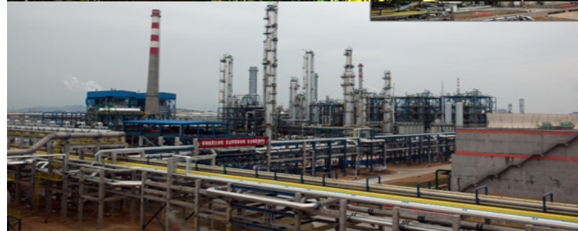
Yangtzi Petro-chemical Plant
